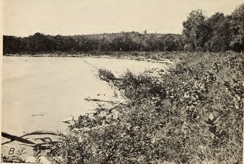
FIGURE 8.—Whole-tree deflector: A , Whole trees placed at toe of bank and cabled to log piles, 1938; B , same bank in 1941, after planting.
